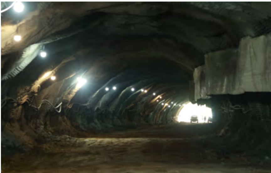
Tunnel construction underway on the North-South Corridor.
